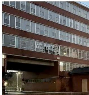
Messages in the windows of Gildengate House tell the story of the impact of closure of the studios
